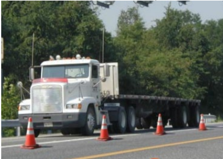
Figure 3: Tractor Trailer Moving on a Shoulder Through a Work Zone 2
