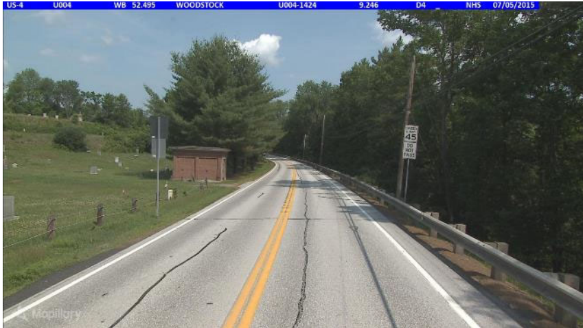
Woodstock, Approaching the right turn at the Hartland Hill Intersection
