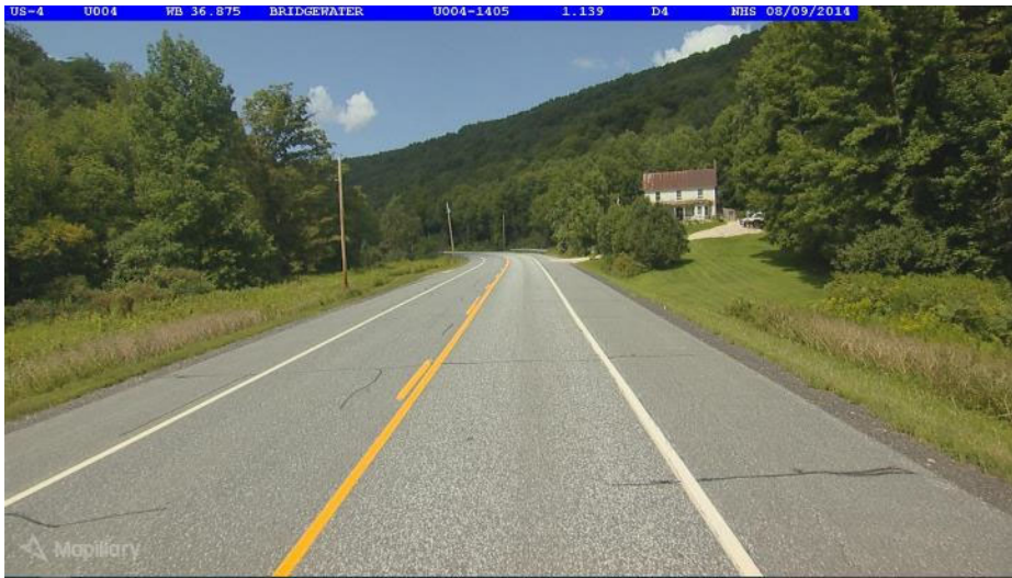
Bridgewater, One mile east of VT 100 South
